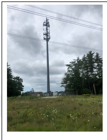
Figure 6 – Southwest View towards Cell Tower (view as of 13/Jul/2021)
